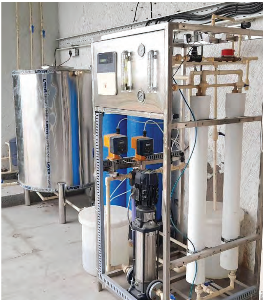
4000 LPD 6 stage Drinking water plant for Amazon Campus, Hyderabad
