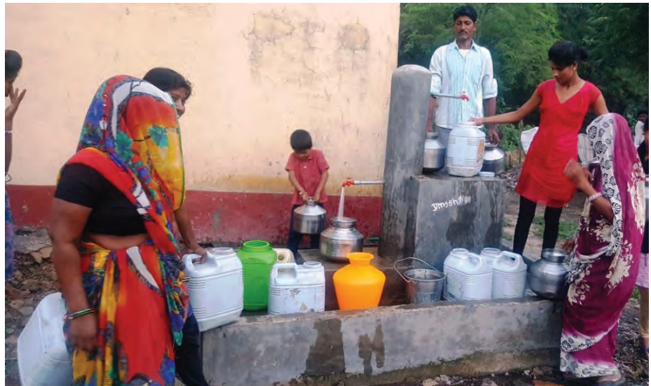
Public Stand Post Water Supply, Gagreen, Rajasthan
